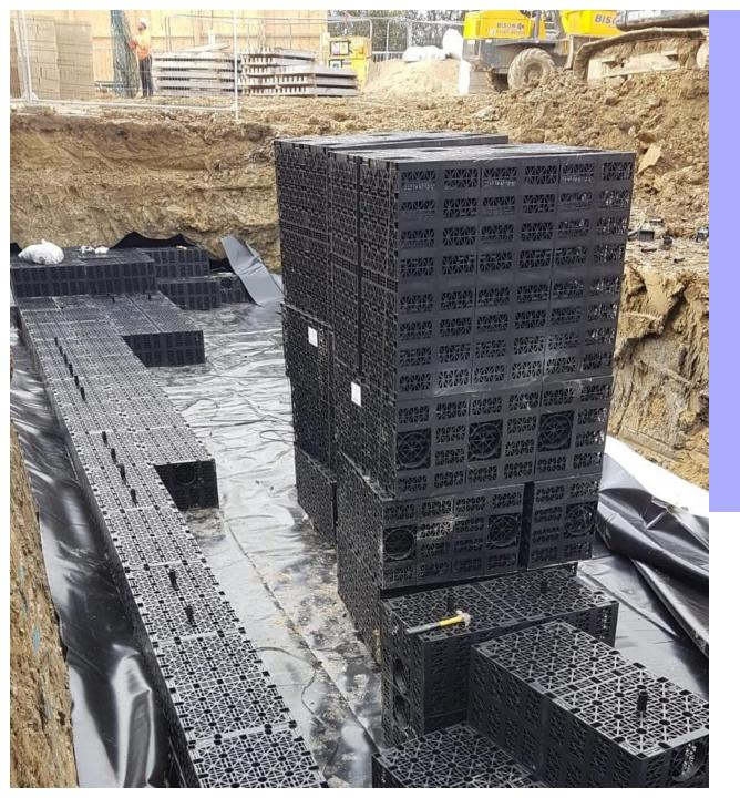
When installing attenuation blocks, we would recommend placing the first initial blocks into an 'L' shape to form structure to the overall shape. Attention must be made to ensure no damage or puncturing to the Geomembrane
