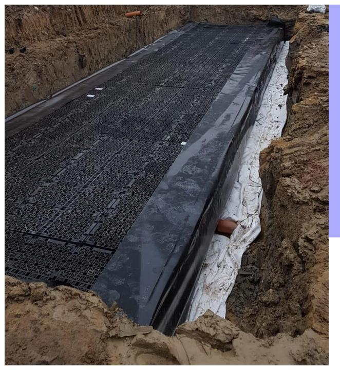
Our Prefabricated Attenuation Tank can now be pulled up and over the formed shape of attenuation blocks.
