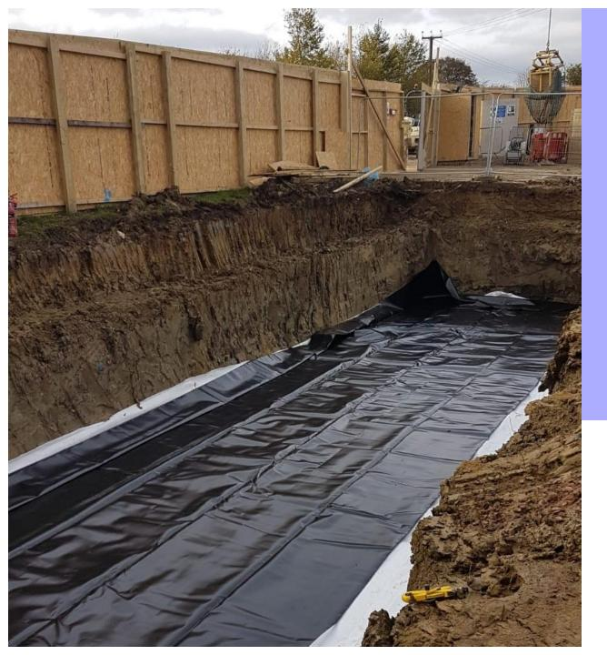
Once the layer of Geotextile has been installed the Geomembrane module can now be positioned and placed on top of the protective fleece layer.
