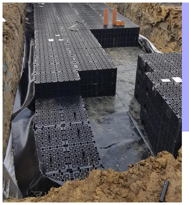
The Attenuation Tank will start to take shape as more blocks are installed.
