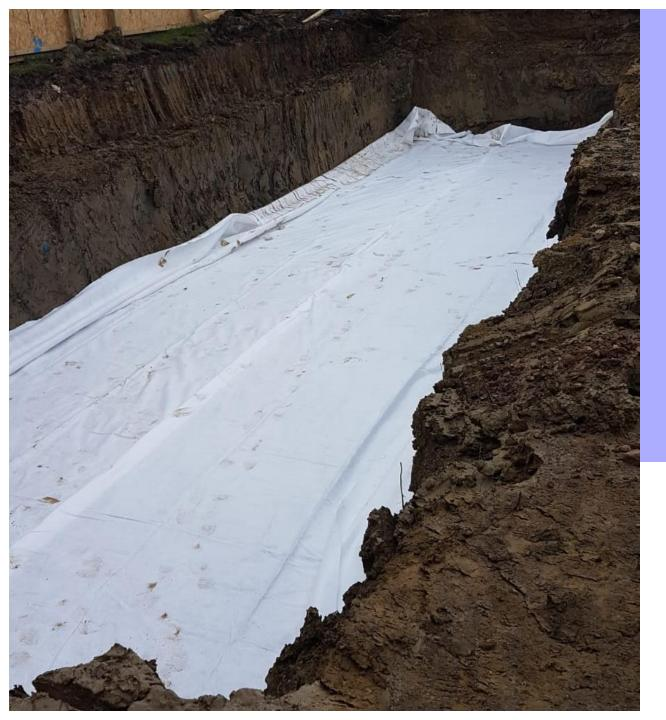
Ensuring the ground is level and free of debris an outer layer of Geotextile Fleece is installed first. This protects the liner from being punctured. Our Geotextile is a high-grade material used for this application offering complete protection to the liner.
