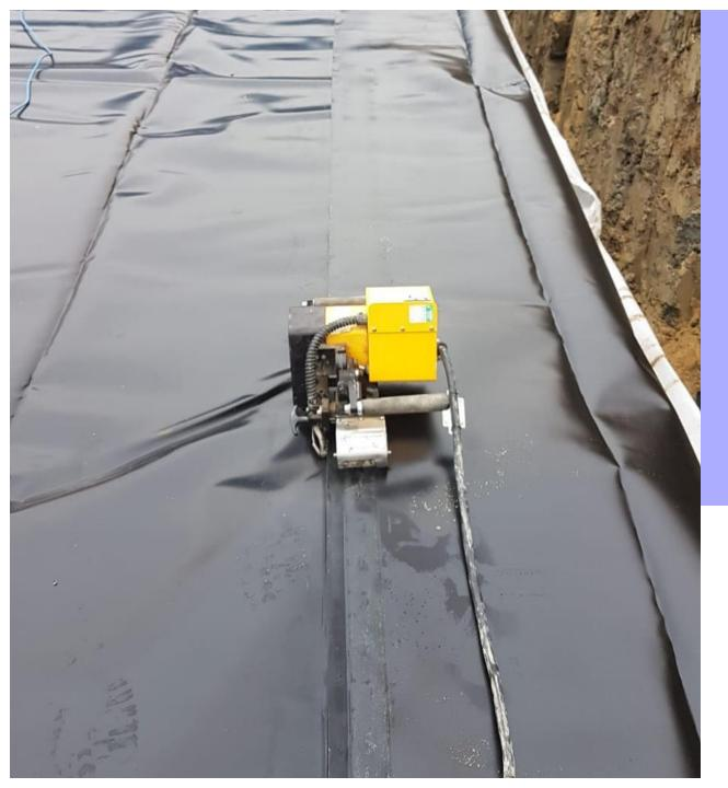
With self installation Attenuation Tanks we provide specialist double sided tape for the installation of the lid. Where required, we can offer skilled technicians to weld the lid liner to the main module, this is priced as an extra charge.
