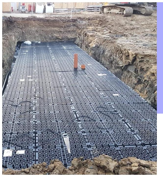
Once all blocks have been placed the next stage is preparing for the installation of the lid
